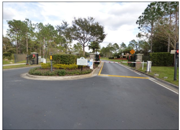
Imperial Oaks Gate System
