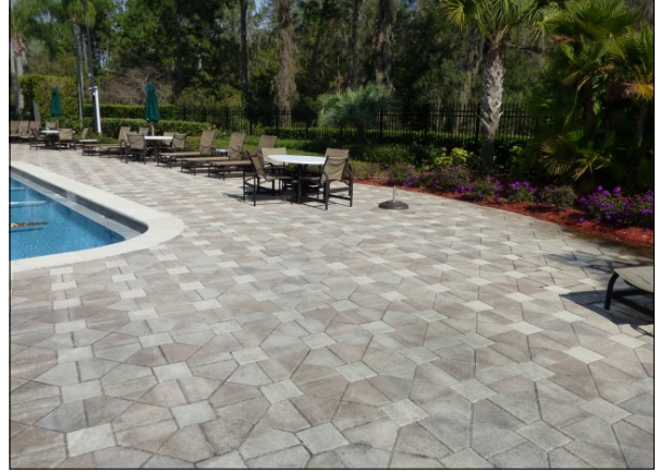
Pool Deck Pavers
